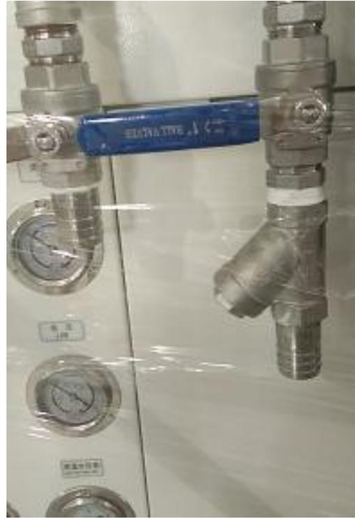
Open the side door of the chiller, and you will see the Y-shaped water filter of the equipment as shown in the picture below
